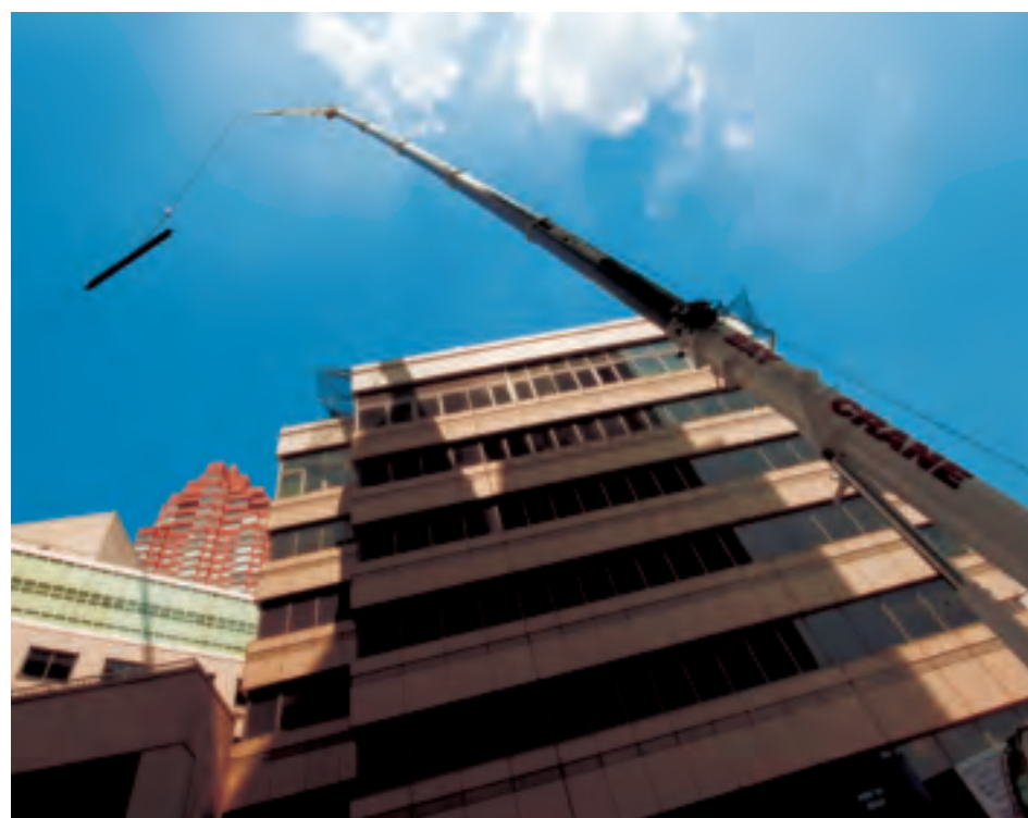
Expansion of the Hospital's East Wing began with the raising of steel this summer.
