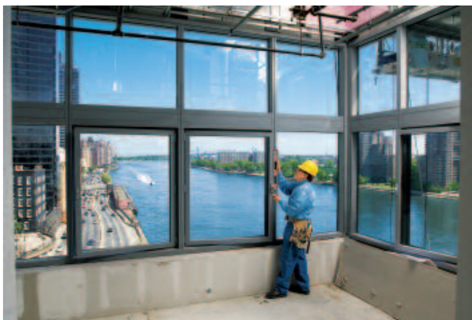
New patient rooms, currently under construction, will overlook the East River.
