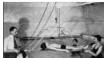
1928 First therapeutic pool in New York City, its unique construction includes a bulkhead with water level above the floor to help facilitate transfer of patients.
